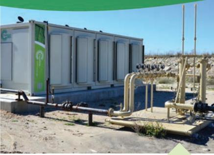
Capstone microturbines in the Eagle Ford Shale Play generate reliable and clean power.
