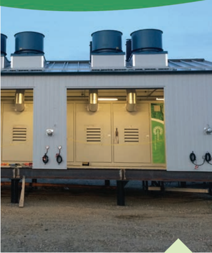
Capstone C800 microturbine at Canadian gas processing facility.
