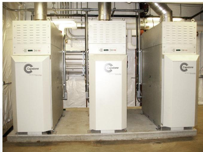
Capstone microturbines at Salem Community College operated continuously during Superstorm Sandy, providing the college and on-campus Red Cross Shelter electricity, heat, and cooling.
