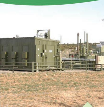
*Eight C65 Capstone microturbines fueled by natural gas direct from the wellhead power this central gathering facility.*
