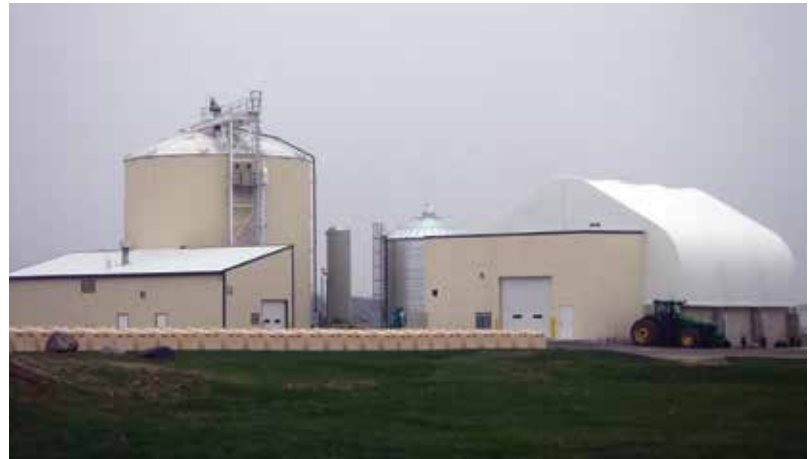
Waste methane gas from the 47-foot-tall anaerobic digester fuels a Capstone microturbine that produces 30kW of clean, green electricity and 45kW of thermal energy used for building heat.
