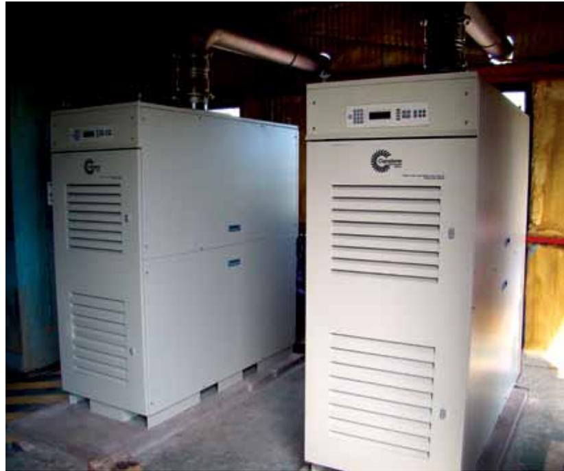
*Eleven Capstone C65 natural-gas microturbines power compressors at this Bolivian pumping station.*
