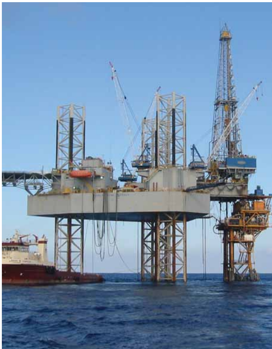
Two Capstone C30, Class I, Division 2 microturbines power this offshore platform in the Gulf of Mexico.
