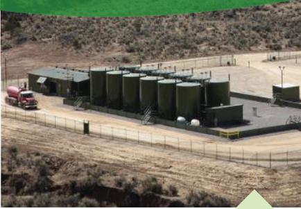
Four C65 Capstone microturbines fueled by wellhead natural gas have averaged 99% runtime since 2011. This is the producer's third microturbine site.
