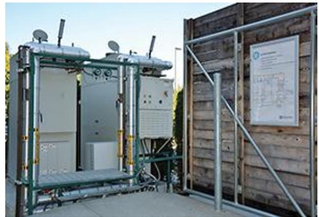
The microgrid at Black & Veatch’s world headquarters includes Capstone microturbines, solar PV, geothermal technology, battery energy storage, and custom controls architecture.
