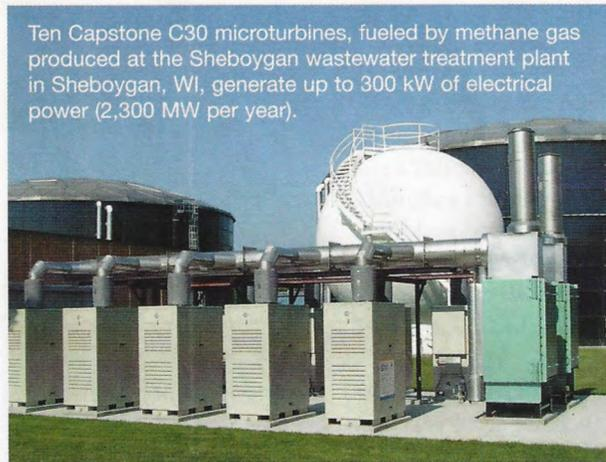
Ten Capstone C30 microturbines, fueled by methane gas produced at the Sheboygan wastewater treatment plant in Sheboygan, WI, generate up to 300 kW of electrical power (2,300 MW per year).
